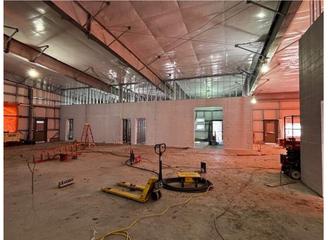
WTP Building Interior Wall Construction
